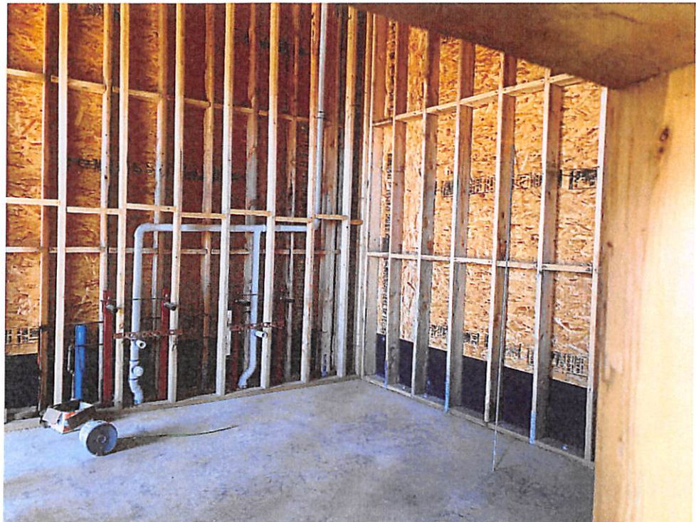
Interior View of the Restroom Building
